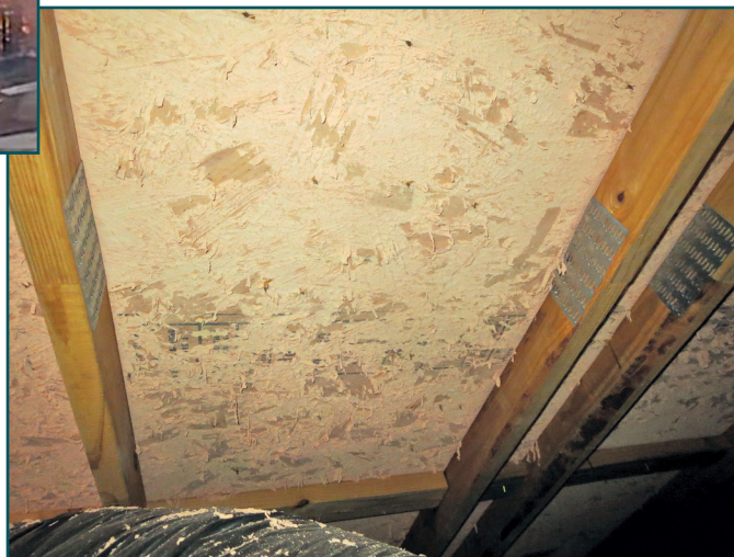
Figure 4 – Failure of fire-resistant paint that was intended to protect a combustible OSB roof deck.
