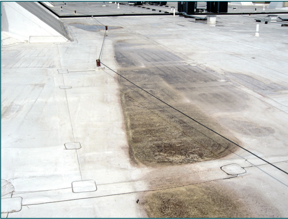
Figure 2 – Typical ponding where the valley of a roof cricket is less than ¼ inch per foot.
