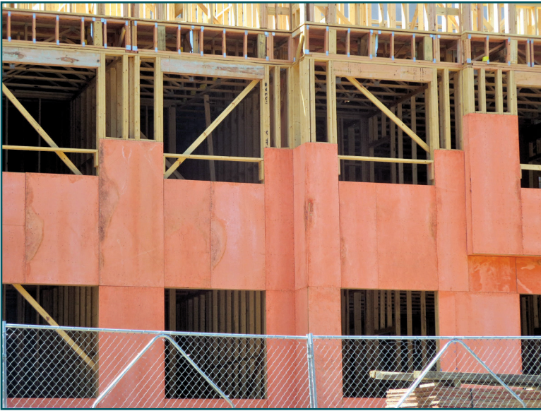
Figure 5 – Water-damaged fire-resistant paint that was intended to protect combustible OSB wall sheathing.
