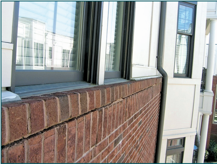
Figure 7 – Brick damage caused by differential building movement.
