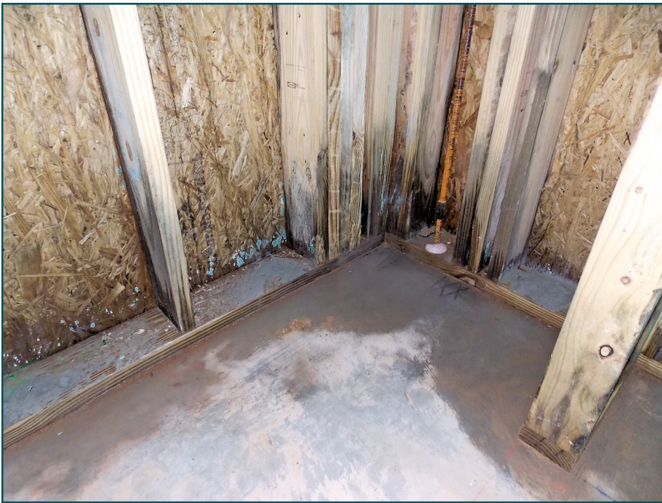
Figure 10 – Water intrusion/damage of a mid-rise wood-frame building under construction.
