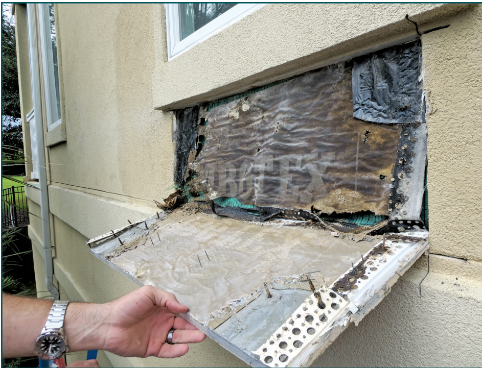
Figure 8 – Moisture damage behind stucco caused by improper integration of two layers of WRB.
