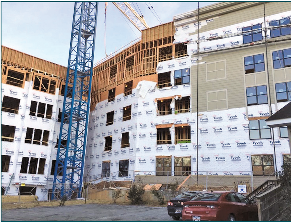
Figure 11 – A haphazard sequencing of multiple trades on the exterior wall of a building under construction.
